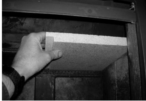
Figure 16 (cont.) - Removing/Replacing the Baffle for Inspection
