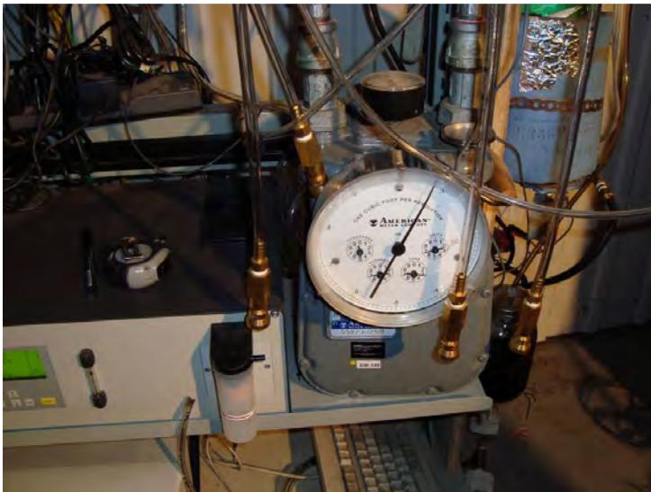
Picture 8: Reference dry gas meter
