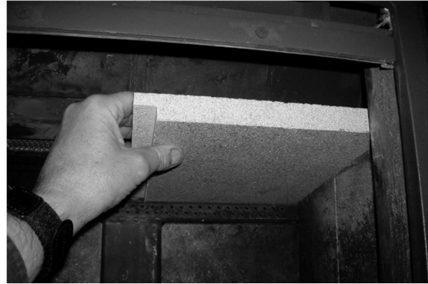
Figure 186 (cont.) - Removing/Replacing the Baffle for Inspection
