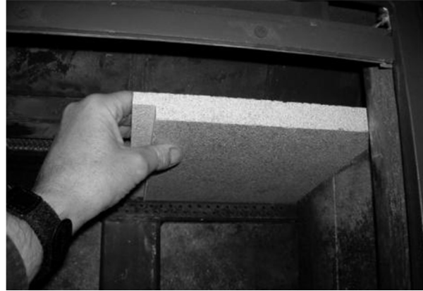
Figure 16 (cont.) - Removing/Replacing the Baffle for Inspection
